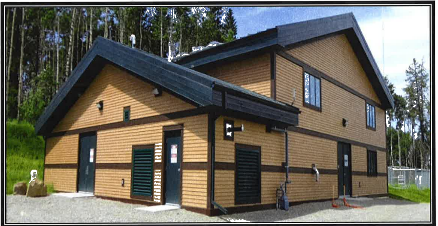
Town of Sundre Water Treatment Plant
