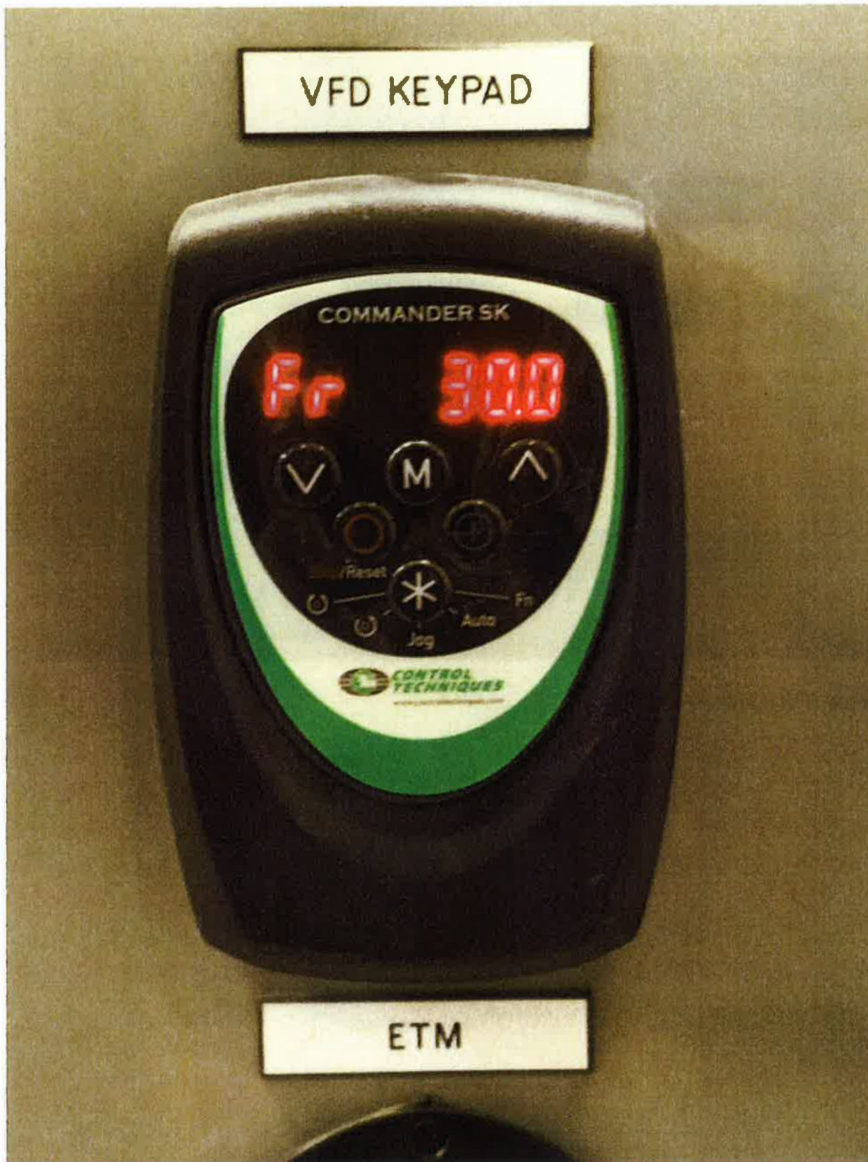
VFD Displaying Frequency for driving pump speed
