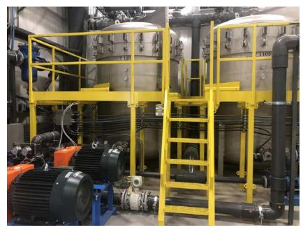
Living Skies electro plate waste removal pumps and filter housing
